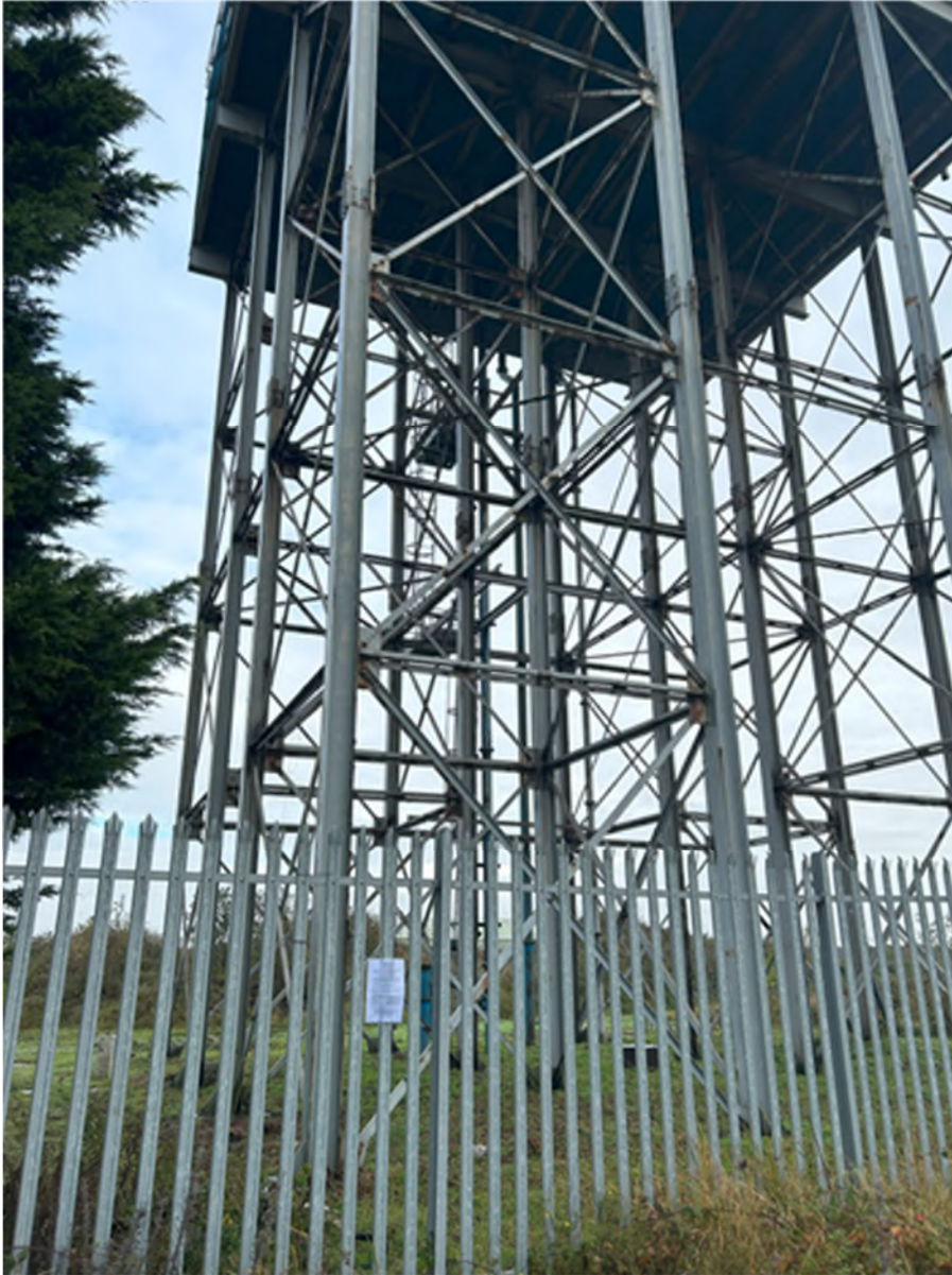
ABP Water Tower
