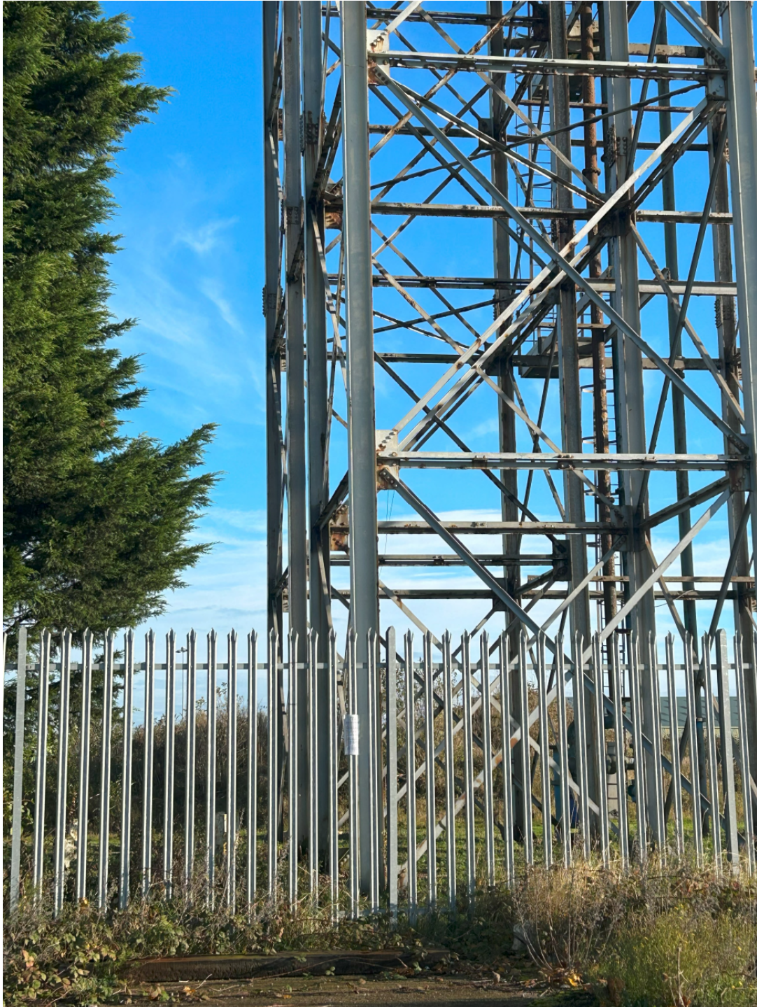
ABP Water Tower
